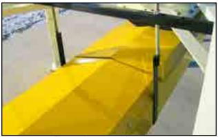
Fig 35 - Install weather covers
