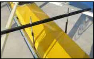
Fig 16 - Hanger bar with brackets bolted on
